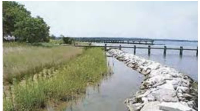
A non-segmented stone sill protecting a marsh habitat. (MD DNR)
