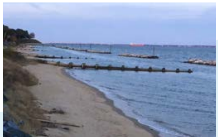
Large off-shore stone breakwater structures paired with timber groins in Anne Arundel county. (Rebecca Swerida)
