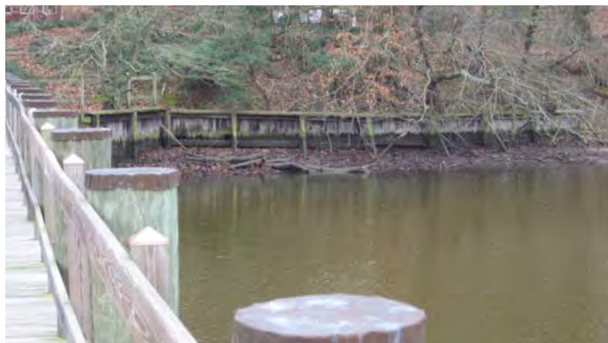
Timber bulkhead with base sediment accumulation visible at low tide in Talbot County. (Rebecca Swerida)
