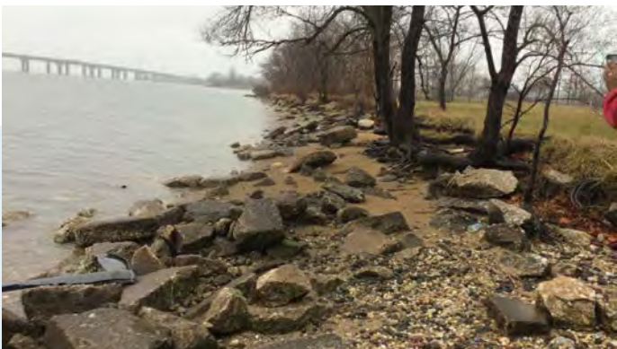
Rubble and loosely placed on-shore stone. (Rebecca Swerida)
